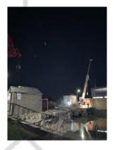
J&M were asked to supply the cranage and Contract Lift for the removal of the Faversham Swing Bridge. On the day, the bridge weighed another 10te due to ballast which had not been accounted for. We supplied a second ATF130G-5 to aid the main crane to lift the bridge out. A great response time with the second crane left a very happy customer.
